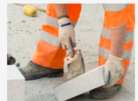
Brush apply tuffbond to the base* and to the underside of the paving units
