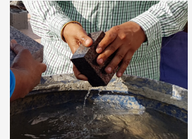
Clean area and underside of paving units
