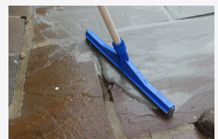
Spread mortar to fill joints and remove excess
