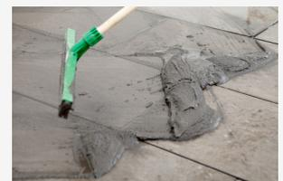
Pour tufftop Utility onto surface and squeegee into joints
